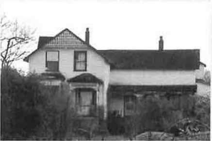
ALEXANDER/GUNN FARMHOUSE 6400 3rd Avenue
