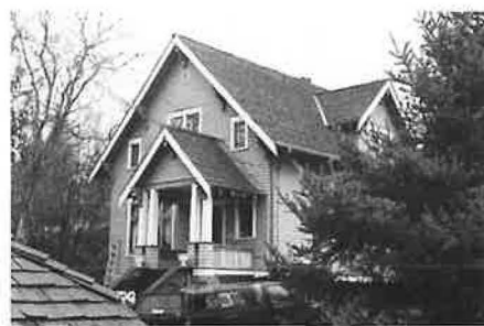
STOKKELAND RESIDENCE 11096 River Road
