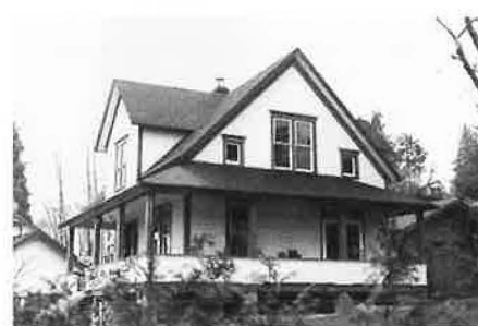
LARSEN RESIDENCE 11102 River Road
