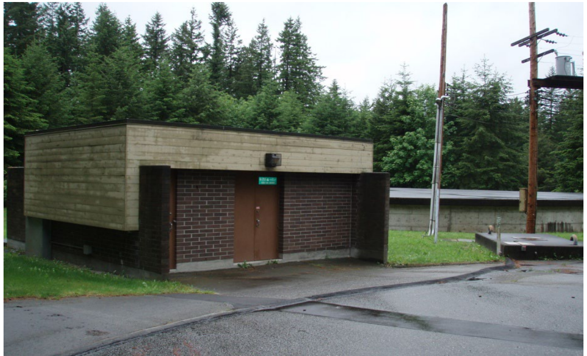
Figure 11: Water reservoir and pump station on 64 Avenue
