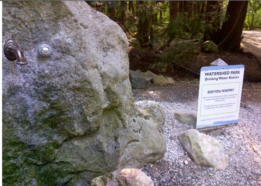
Figure 20: Watershed Park Drinking Water Station, constructed 2012
