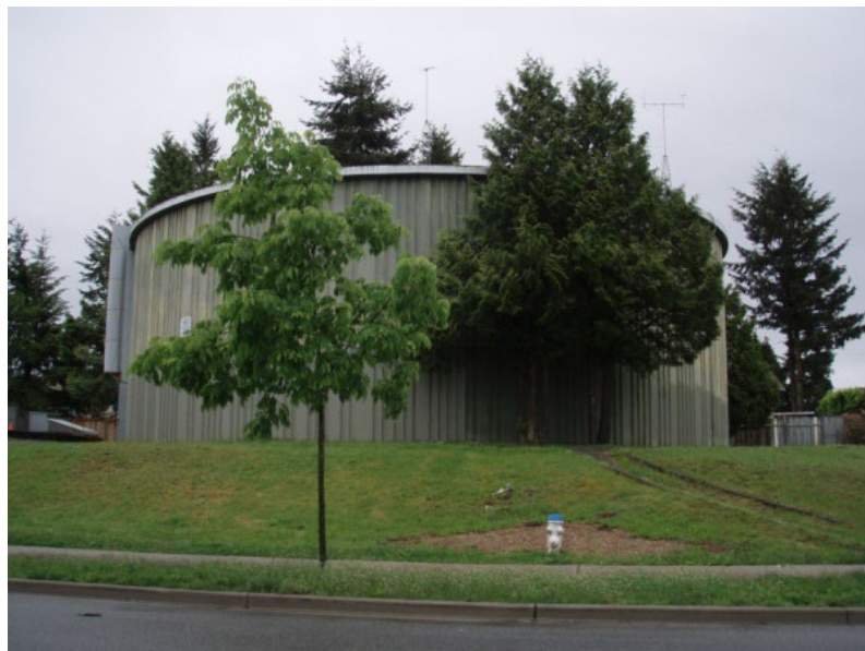
Figure 16: Hellings Reservoir in North Delta
